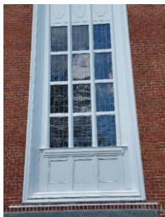
After repairs (new clear glass)
