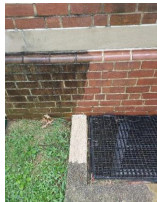
BEFORE AND AFTER CLEANING/POWER WASHING.
